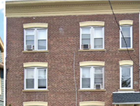
FAIRFIELD AVENUE STAMFORD OPENED: 2019 FAMILY UNITS: 3
