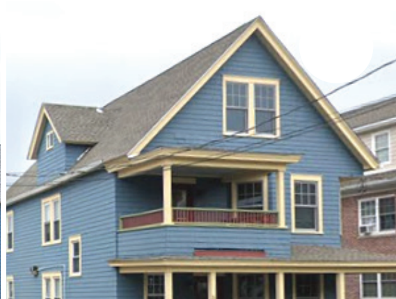
FAIRFIELD AVENUE STAMFORD OPENED: 2024 FAMILY UNITS: 4
