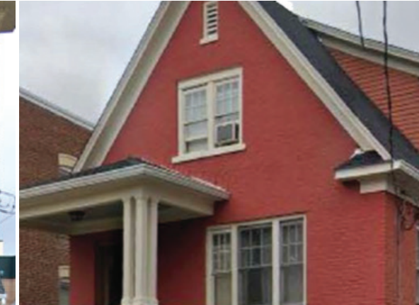
FAIRFIELD AVENUE STAMFORD OPENED: 2019 FAMILY UNITS: 5
