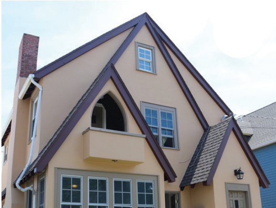
FAIRFIELD AVENUE STAMFORD OPENED: 2019 FAMILY UNITS:3
