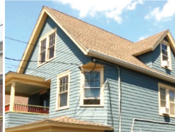
FAIRFIELD AVENUE STAMFORD OPENED: 2019 FAMILY UNITS: 4
